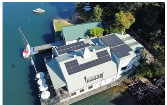
Our newly installed solar panels
